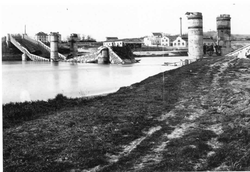
Plate 108 Photograph of the Argenteuil railroad bridge destroyed during the Franco-Prussian War, c.1870–71. Photo: Roger Viollet, Paris.
